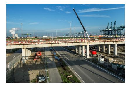
Construction of a Truck Bridge over St Antoniusweg at the Deurganckdok on the Left Bank/Antwerp. The Truck Bridge was built on the site of MSC PSA European terminal, but extends over the public domain. The bridge has a length of 77m and a width of 12m.
