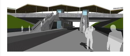
The existing accesses (concrete stairs and escalators) to the platforms in Antwerp South station will be demolished and replaced by a bicycle lift and precast concrete stairs.
