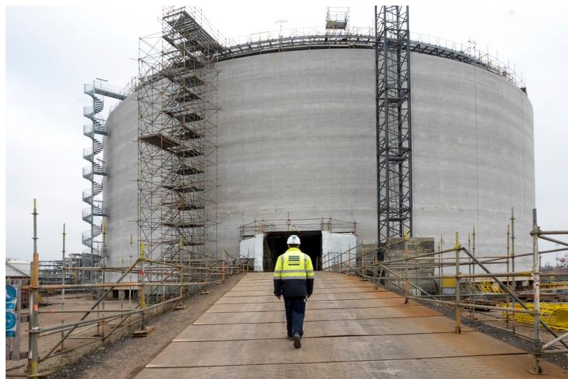
Franki Construct built an ammonia tank on the BASF site in the port of Antwerp for the German petroleum & gas engineering company, SPG Steiner. The tank's diameter is 72 m, and it is more than 26 m high. The 26-m high concrete wall was erected in a continuous 24-hour shift system using sliding formwork.
