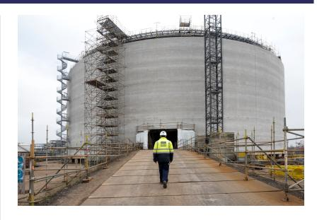
Franki Construct built an ammonia tank on the BASF site in the port of Antwerp for the German petroleum & gas engineering company, SPG Steiner. The tank's diameter is 72 m, and it is more than 26 m high. The 26-m high concrete wall was erected in a continuous 24-hour shift system using sliding formwork.
