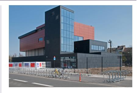
Construction of a signalling centre for the Belgian railways and demolition of an existing post office building. The complete building forms a Faraday cage to protect the railway signalling. This was accomplished by earthing 4,100 m² of concrete walls and interconnecting all concrete reinforcement.
