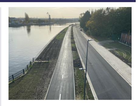
Between Grimbergen and Vilvoorde, we are constructing the 'Noordkanaalfietsroute', a safe and fast cycle route that is part of the F23 cycle route between Boom and Brussels. We are responsible for the entire route, for the road and sewerage works and for the construction of the cycle route. In Vilvoorde, we built a 150-metre quay wall as part of the same project.
