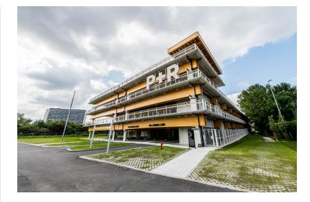
This ultramodern 'park and ride' car park (12,000 m<sup>2</sup>) in Merksem has room for 690 cars and 150 bicycles and 18 charging points for electric vehicles. The building is characterised by its light and open construction, in which wooden beams play the main role.
