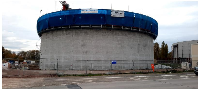
Construction of a cylindrical concrete drinking water reservoir with an inner diameter of 38.4 m, a wall (via sliding formwork) with a thickness of 45 cm and a height of 16.5 m, including surrounding construction.
