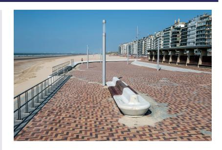
The seawall in Wenduine has been completely demolished and rebuilt according to a new concept. The sea dyke is now safer, wider and more attractive. Two storm walls were placed on the new and stabilised dyke body to stop waves from overtopping. One wall - a secant wall topped by a parapet of exposed concrete - slopes towards the beach. The second parapet (landward) is shaped like a bank and was also built on top of a secant wall.
