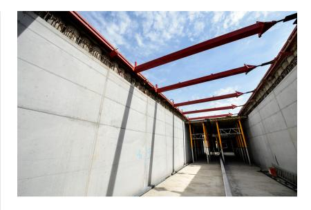
Storm water reservoirs connected to the drainage system that can collect 10,000 m<sup>3</sup> of water during heavy storms, relieving the pressure on sewers. Buffered water is discharged into one of the main collectors in Brussels, half using a gravitational outlet, the other half using pumps.
