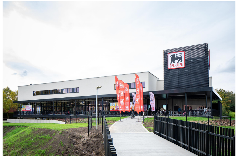
Construction of a supermarket for Delhaize.
