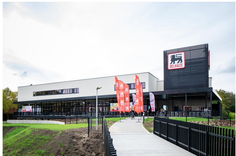
Construction of a supermarket for Delhaize.
