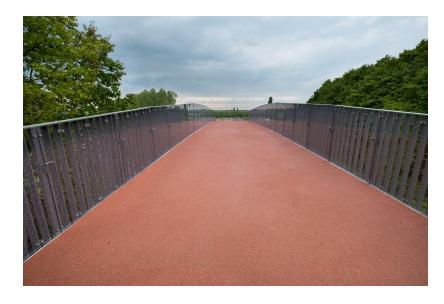
The longest composite bridge in the country was installed on the border between Boechout and Mortsel. It is the first bicycle bridge made from fibre-glass-reinforced plastic, and it has the largest free span of its kind in Belgium. This is a first on the F11 Antwerp-Lier bicycle highway. The bridge was put in place in one piece (5 m wide and 30 m long), and it only weighs 33 tonnes. Hoisting was carried out using a 400-tonne mobile crane with a span lift.
