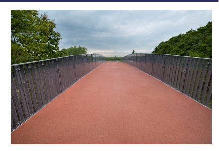
The longest composite bridge in the country was installed on the border between Boechout and Mortsel. It is the first bicycle bridge made from fibre-glass-reinforced plastic, and it has the largest free span of its kind in Belgium. This is a first on the F11 Antwerp-Lier bicycle highway. The bridge was put in place in one piece (5 m wide and 30 m long), and it only weighs 33 tonnes. Hoisting was carried out using a 400-tonne mobile crane with a span lift.
