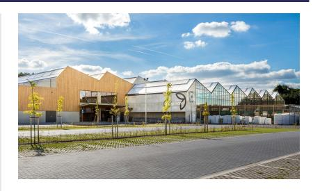
Oh'Green's new site in Aarschot is a pilot shop of Garden Center Holding. Cosimco was responsible for its construction on a site of just over 44,000 m². Due to the conditions imposed by the PRUP, the building was designed lengthwise, parallel to the Diestsesteenweg. Due to the steeply sloping terrain in the first 50 metres from the street, the garden centre was built half underground.
