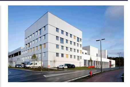
This brand new fire station is one of the most important stations in the region. The station has a five-storey office building and a vehicle hall with a full span. This means that there are no propping poles that could impede a rapid response. On top of the hall there is a fitness room and a sports hall. The new building also has sleeping quarters, workshops, an exercise tower and an exercise ground. By the way, the whole building is almost energy neutral.
