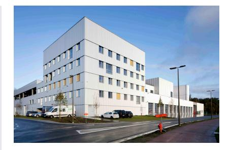
This brand new fire station is one of the most important stations in the region. The station has a five-storey office building and a vehicle hall with a full span. This means that there are no propping poles that could impede a rapid response. On top of the hall there is a fitness room and a sports hall. The new building also has sleeping quarters, workshops, an exercise tower and an exercise ground. By the way, the whole building is almost energy neutral.
