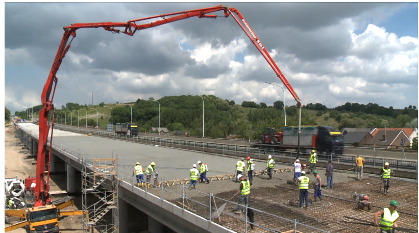
Rebuilding of the A13 motorway viaduct at Bassenge (Boirs).
