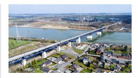
The 523 meter long Pont des Allemands, in use since 1917, is one of the most remarkable works of art on the Belgian railway network. Every day, about 80 freight trains use it to cross the Meuse. A century after its construction, the viaduct was due for a rejuvenation. As part of a complete renovation of this viaduct, we installed a new bridge deck, among other things. The tracks and overhead lines were also renewed and the eight concrete piers were reinforced.
