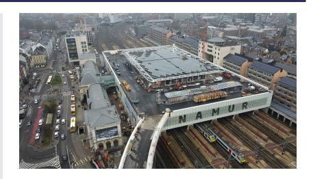
Namur station – building the Multimodal Station. Phase II: Construction of the coach station, its access and associated road works.
